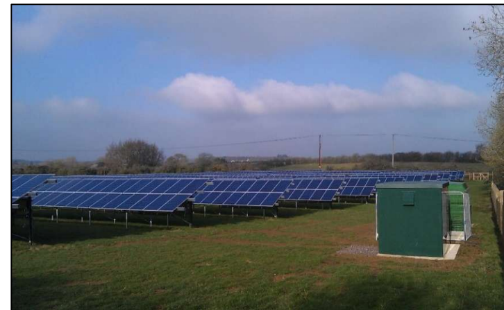
Figure 3.2: Ground mounted PV panels and transformer
